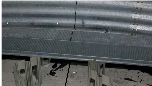
Image 4 – Marking bin wall, installing first plank
