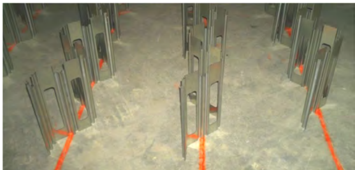
Image 3 – Positioning SuperWave Supports
