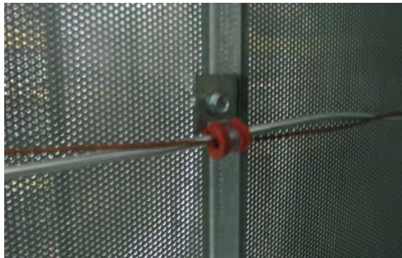
Image 4-32 – RTD Temp sensor wire
