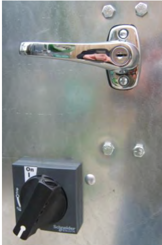
Image 20 – Latch and switch in “Off” position
