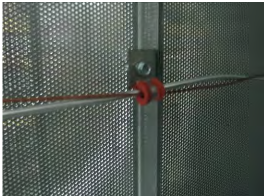
Image 11 – Plenum RTD and over-temp capillary
