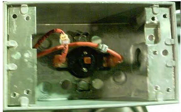
Image 4-6 - Vapor Over-Temp Switch
