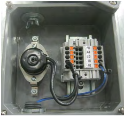
Image 4-8 – Grain column over-temperature switch
