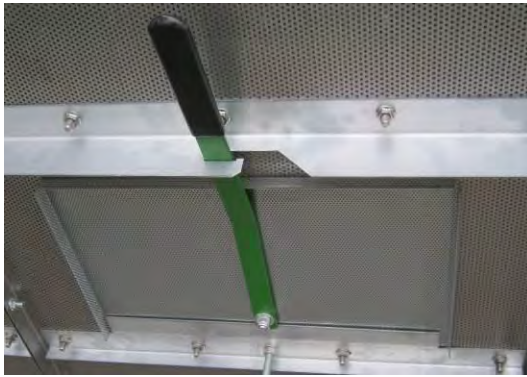
Image 26 – Cleanout/inspection door
